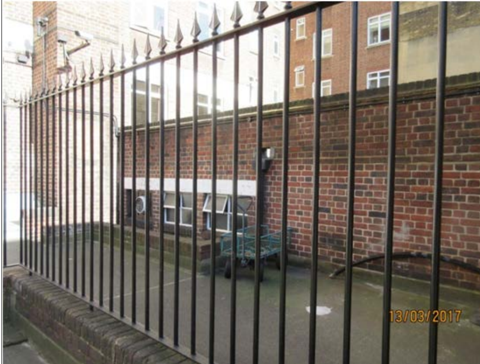
North-west elevations of Sussex Lodge boiler room
