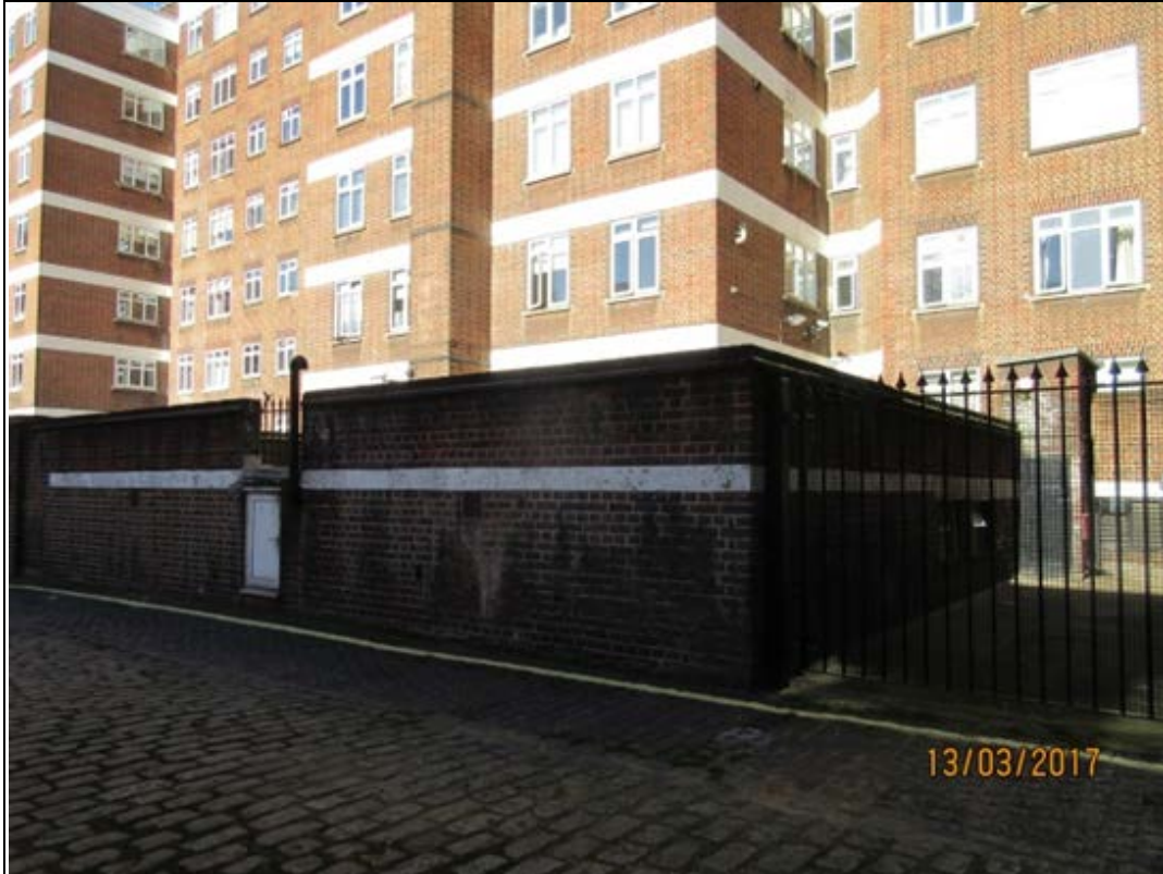
Existing boiler room building
