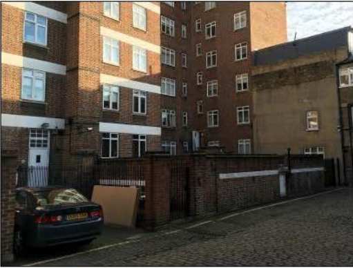
15 VIEW OF BOILER HOUSE
